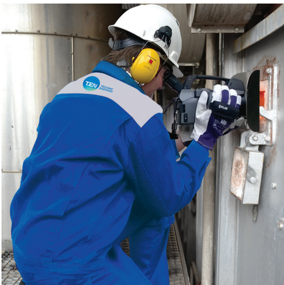
The quick assessment is done with data provided by an infrared camera.
